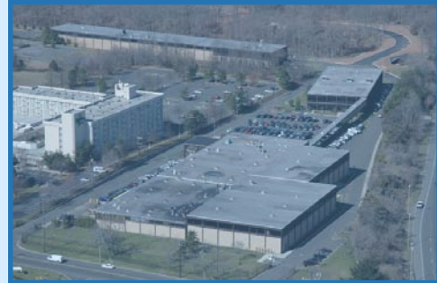
Aerial view of Rotor Clip Company, Inc. Somerset, NJ
